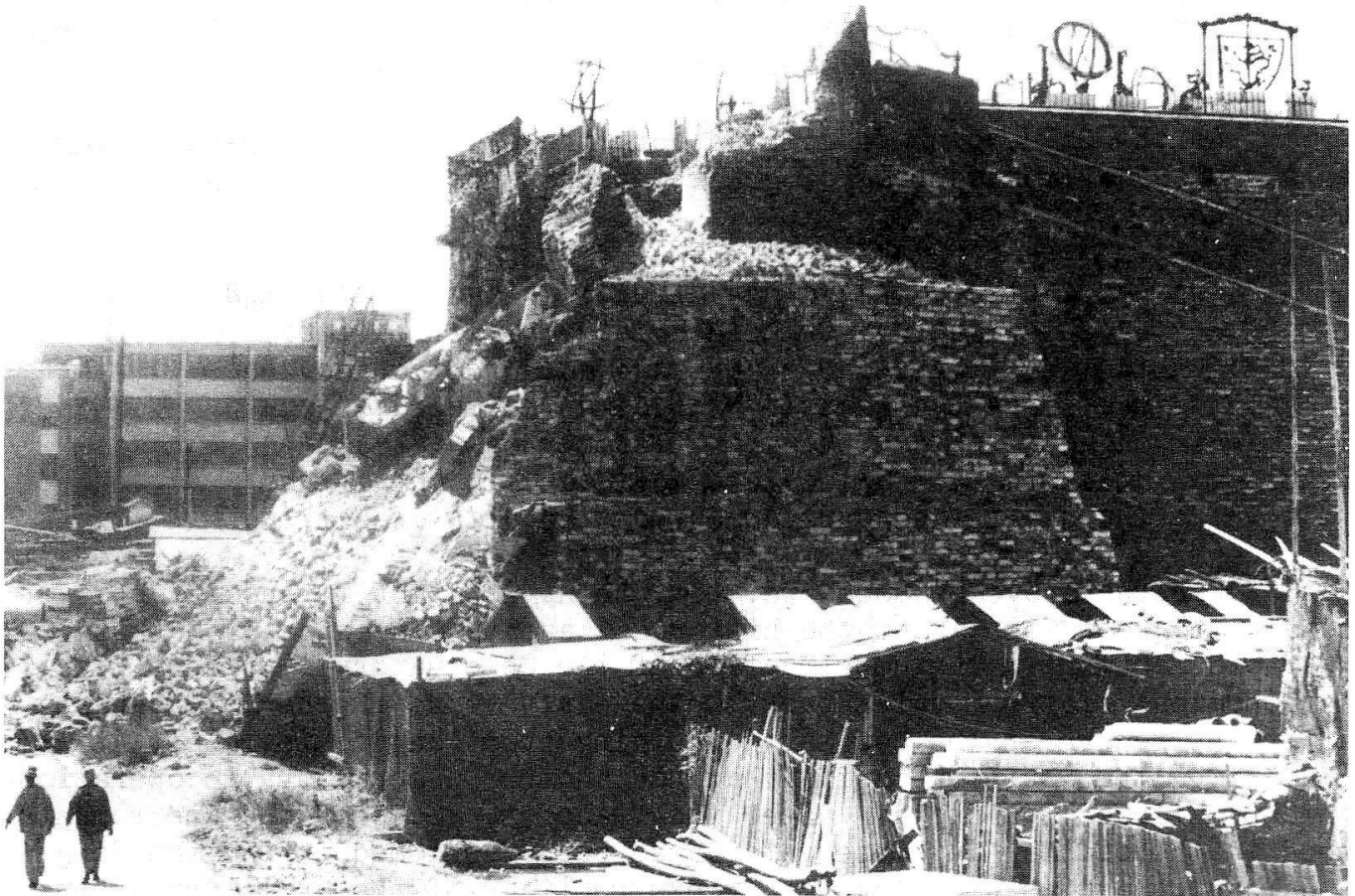
THE ASTRONOMICAL OBSERVATORY'S PLATFORM PARTLY COLLAPSED AFTER A RAIN STORM
